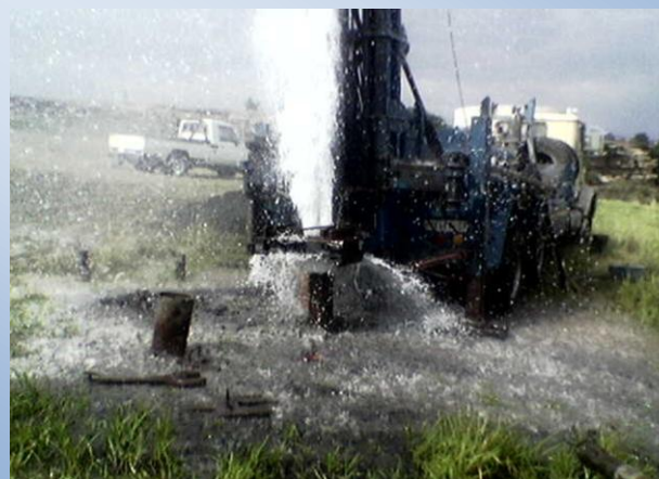
Water strike while drilling
